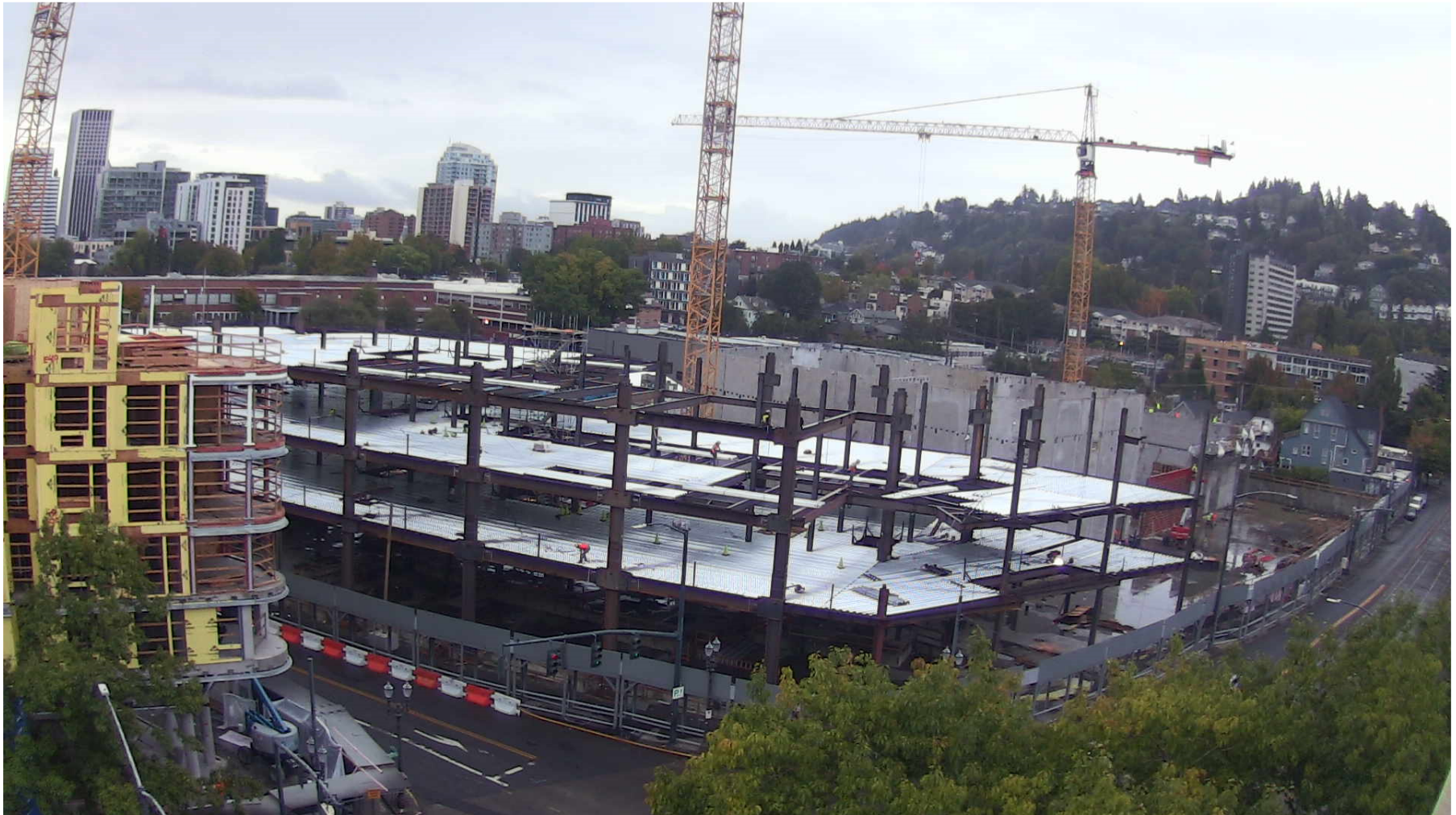
Site photo – Oct. 14, 2020
