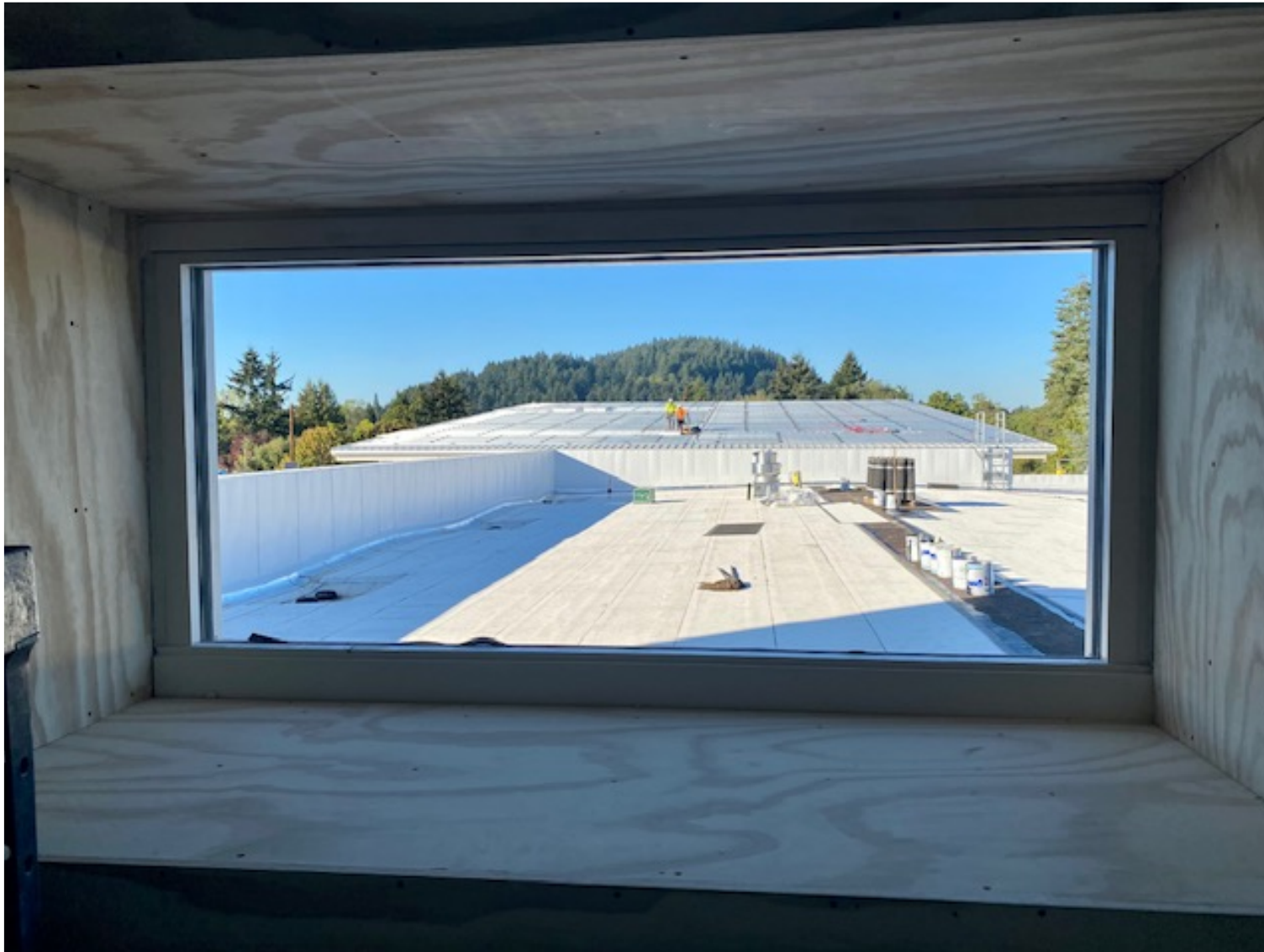
View of Roof & Solar PV Array / October, 2020
