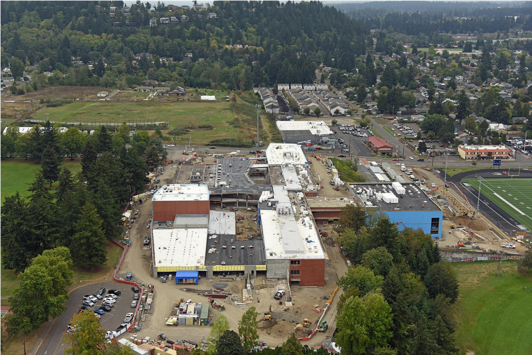
Aerial photo – October 8, 2020
