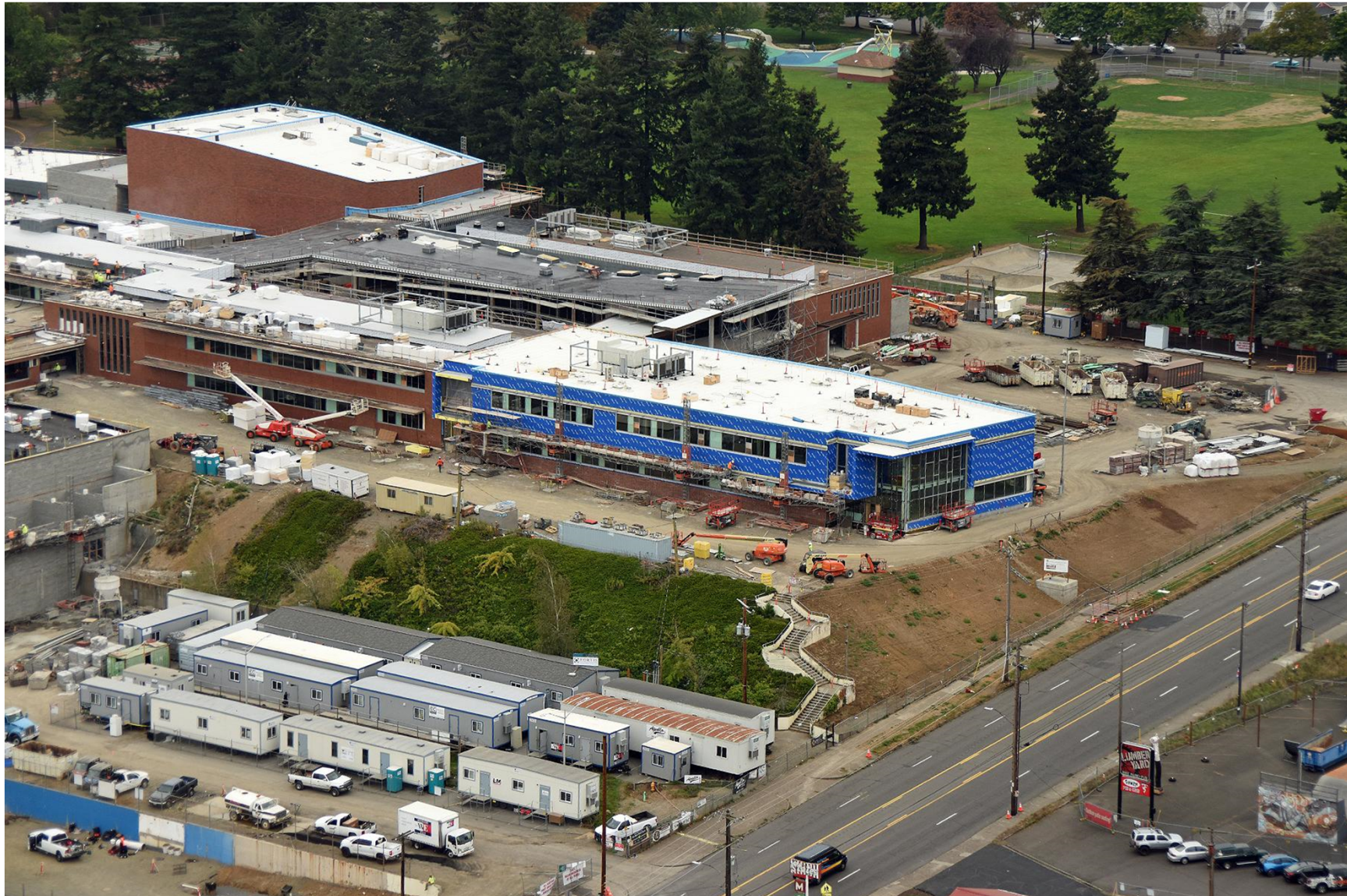
Aerial photo – October 8, 2020
