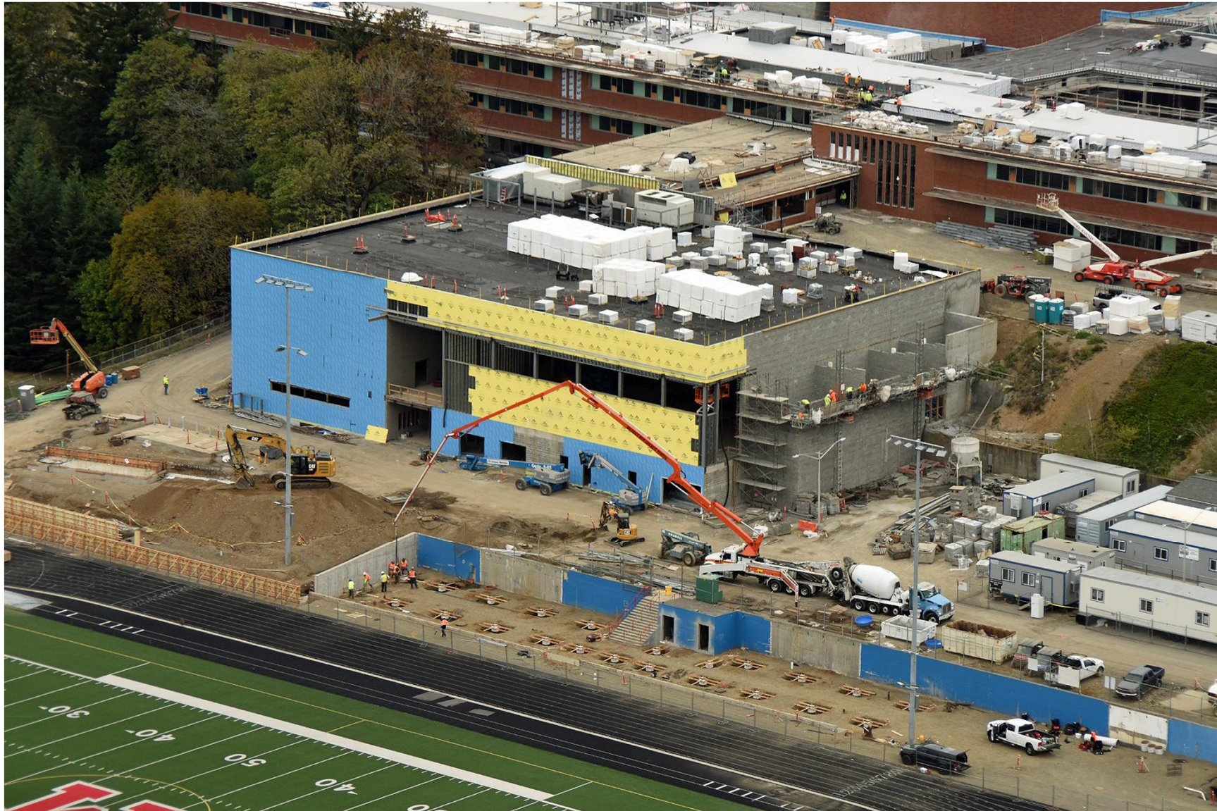
Aerial photo – October 8, 2020
