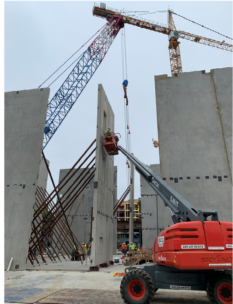
Tilt Panels of the auditorium shell.
