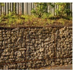
Gabion Retaining Wall
