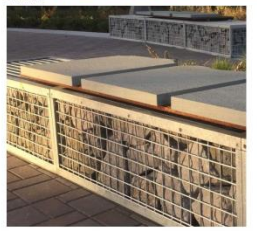
Gabion Retaining Wall
