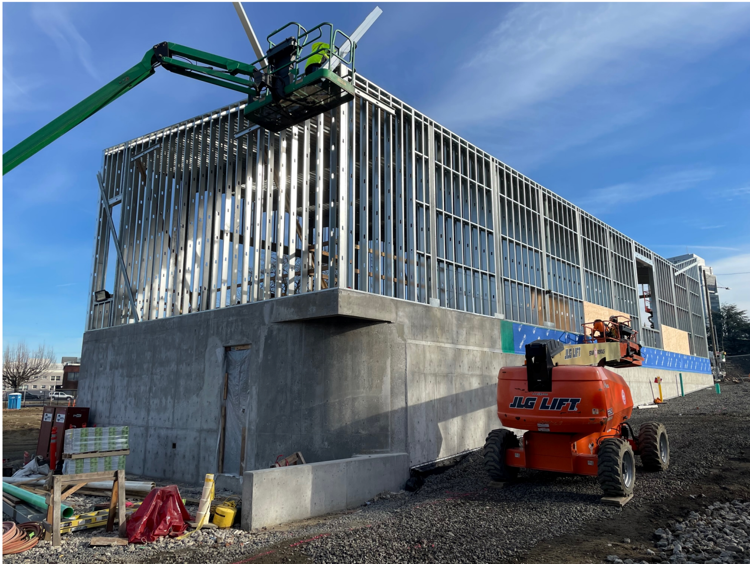
Field Service Building
