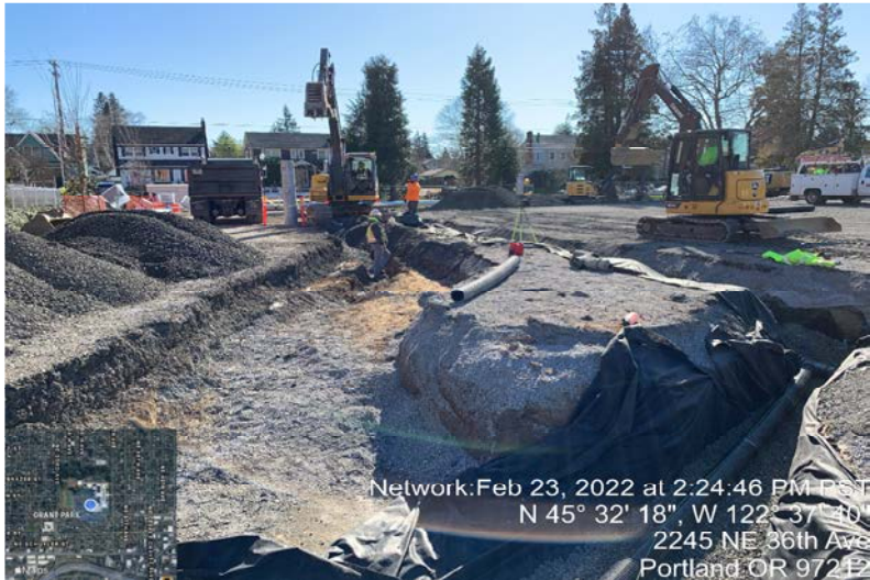
Installation of new field drainage in southeast corner
