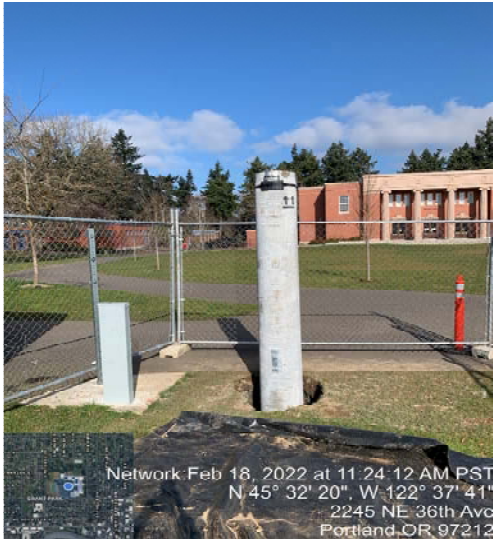
Typical field light base installed
