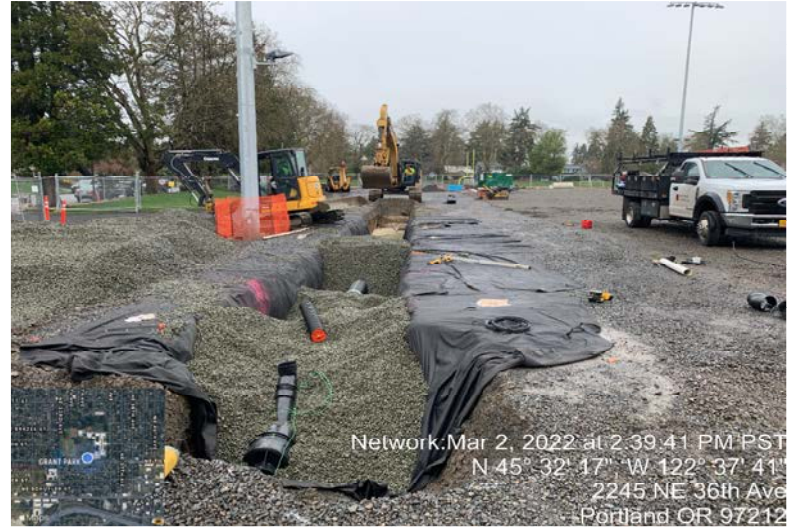
Installation of detention trench and pipe on south field edge
