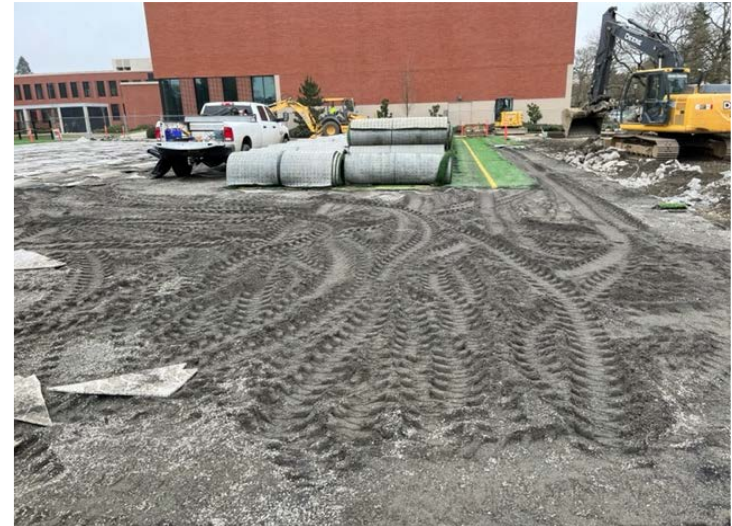
Rolls of removed artificial turf prepped for removal and recycling
