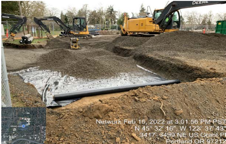
Installing and compacting base rock subgrade for asphalt paths on south end
