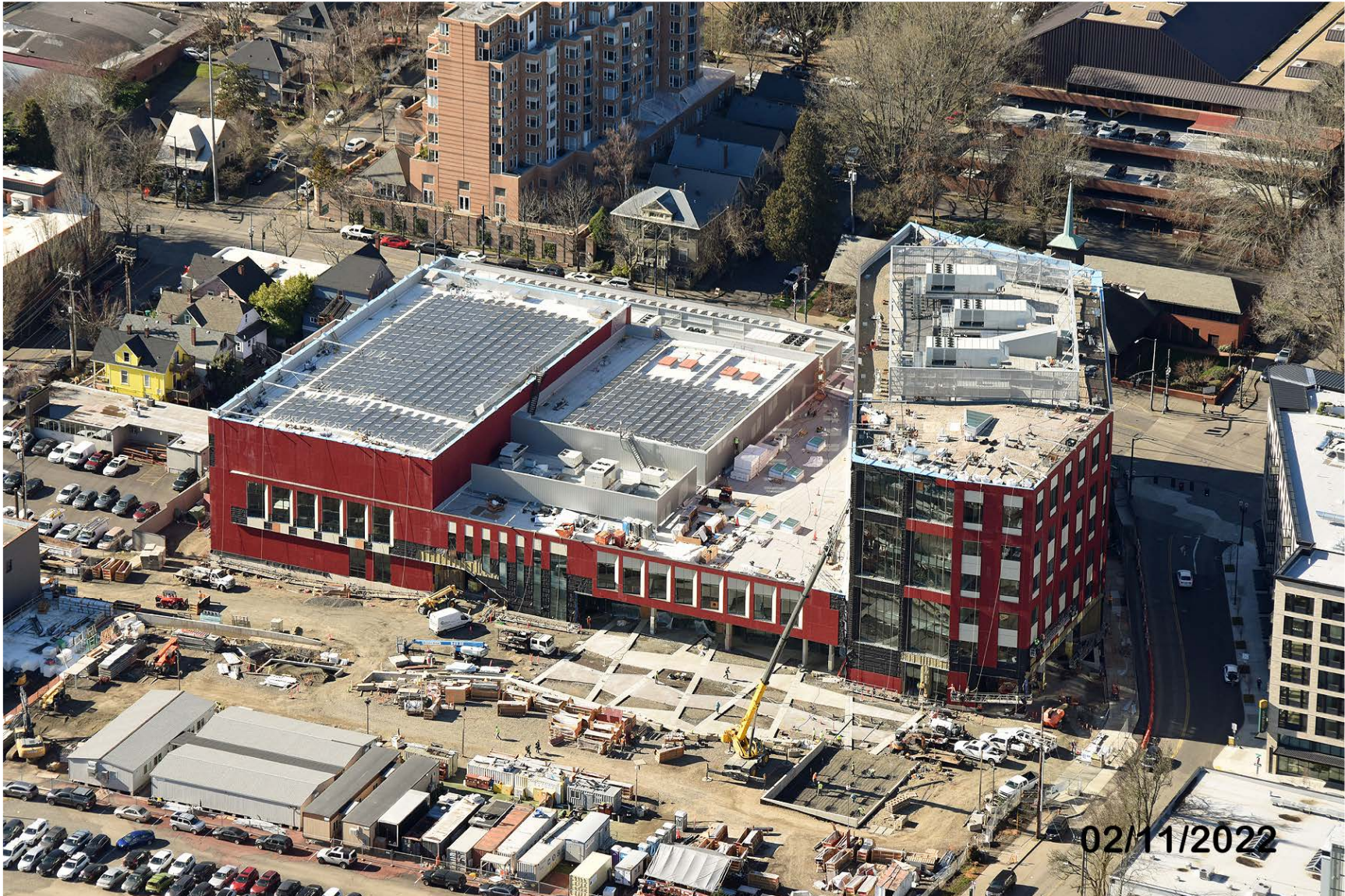
Aerial photo – February 11, 2022
