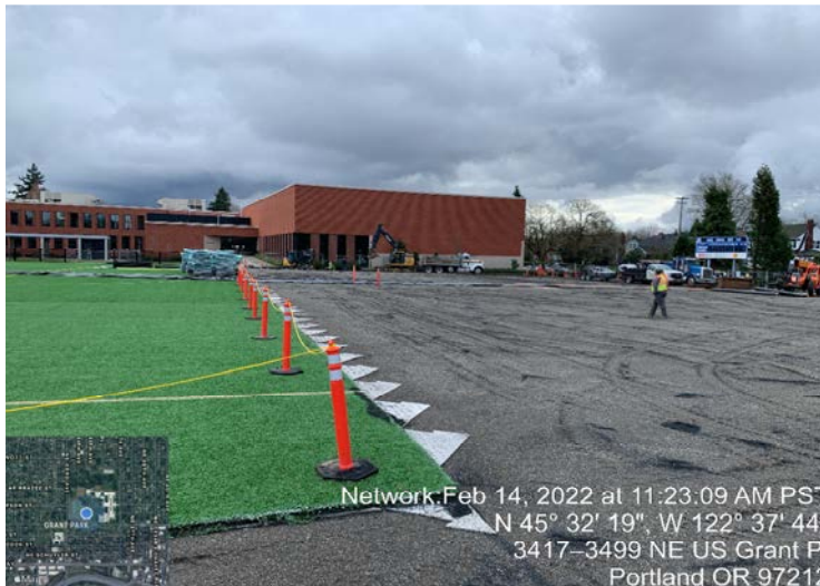
Existing turf and shock pad removed on south end
