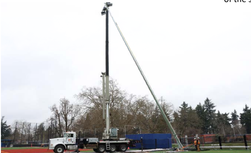
Crane truck lifting field light poles into place
