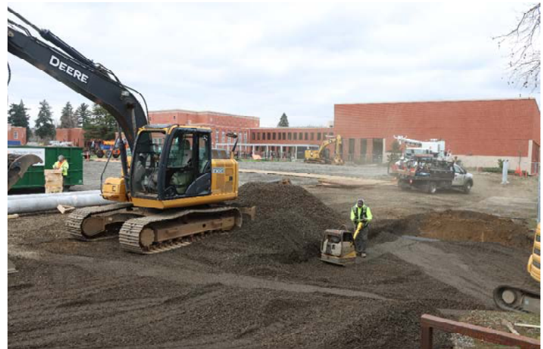
Installing and compacting base rock subgrade for asphalt paths on south end
