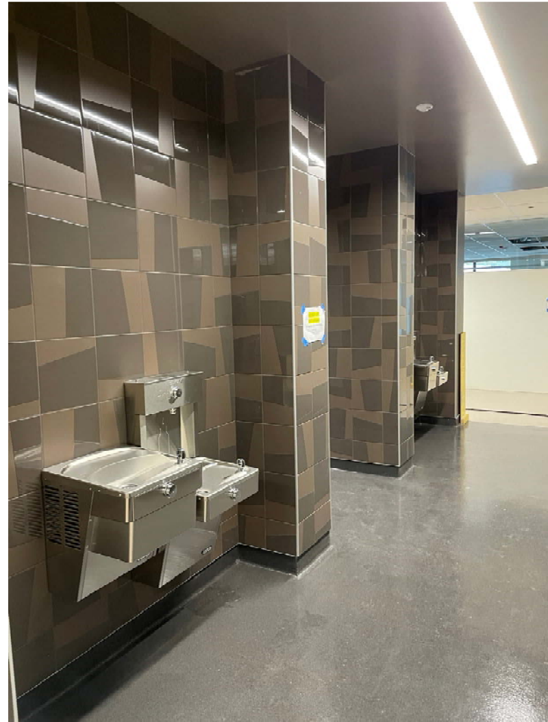
Restroom Tile and Fountains
