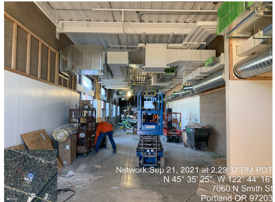
Looking inside CTE space under construction, from the west.
