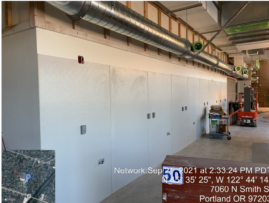
Build-out of teaching wall inside CTE space.
