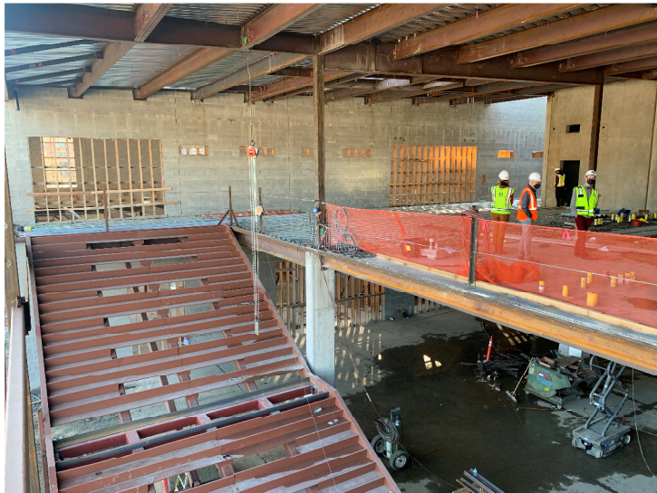
Steel stairs leading to the gym
