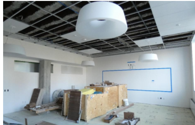
Mock Up Classroom
