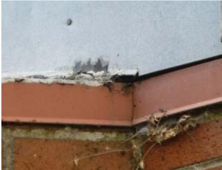
Flashing at intersection of metal panel to top of wall
