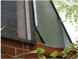
Flashing failure at window to metal panel siding and to of brick wall
