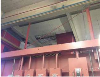
Example of ceiling damage from water intrusion, and typical acoustical panels
