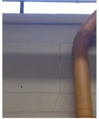
Cracking at interior side of exterior wall,typ.
