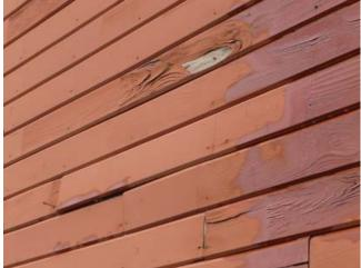
Deterioration at wood siding
