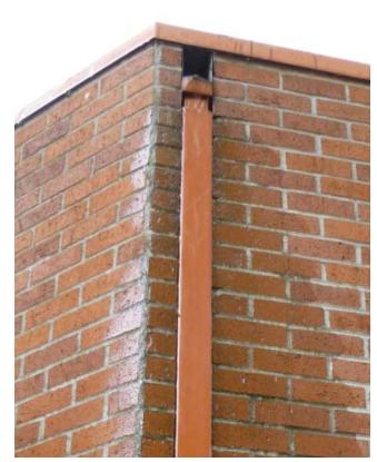
Unsealed wall pentration and water overflow at conductor head
