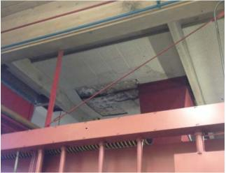
Ceiling failure due to water infiltration
