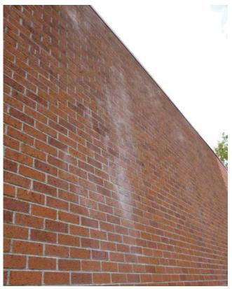
Efflorescence at brick veneer wall, typ.
