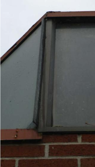
Metal panel to aluminum window and top of wall intersection
