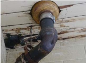
Roof deck detoriation at drainpipe
