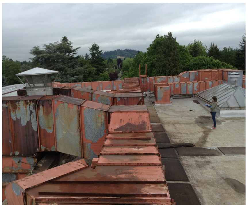
Existing Roof and Rooftop Mechanical System
