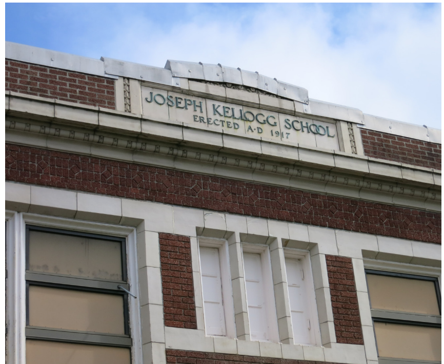
Existing Main Building Parapet Coping and Windows
