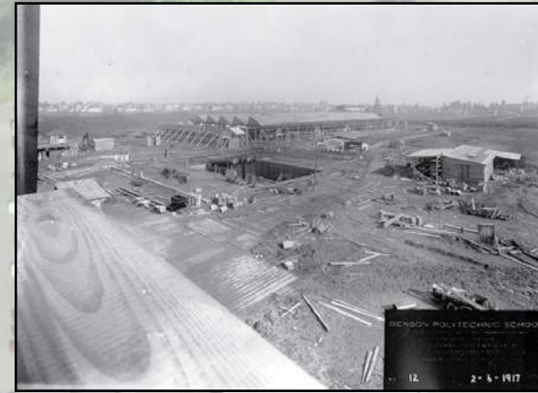
Construction of Benson High School Industrial Arts Building from scaffolding of first unit, looking northeast, 1917.
