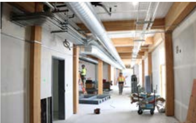
hayu alqi uyxat - Hallway Interior Finishes and Installs, February 22, 2024
