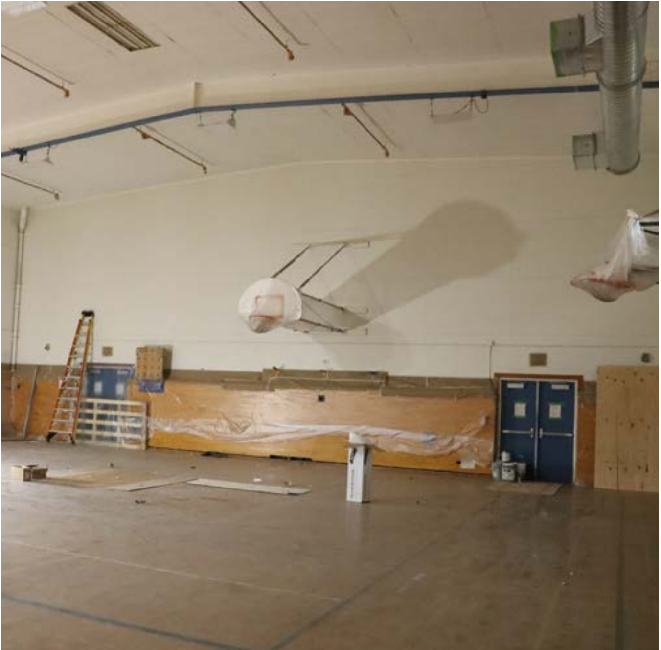
Harrison Park Middle School - Gym Construction, March 4, 2024
