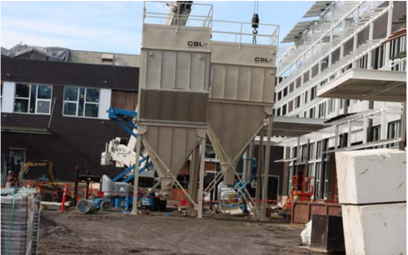
Benson High School - Dust Collector Crane Install, February 22, 2024
