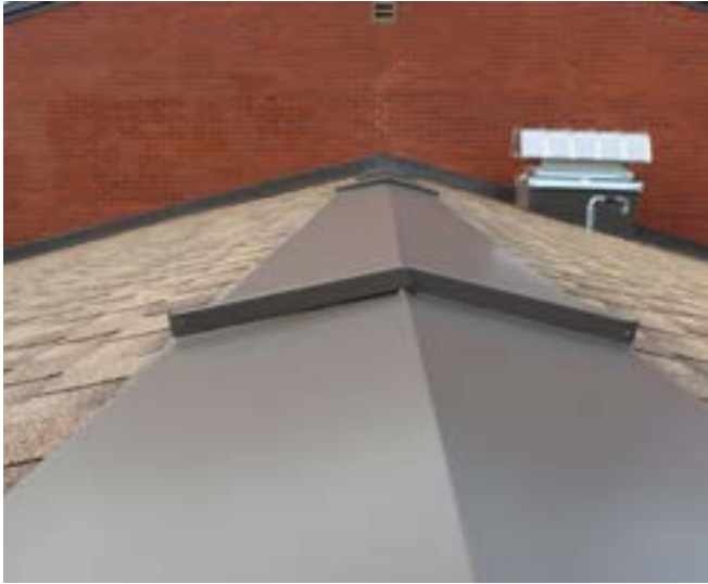
Markham Elementary School - New Roof, December 18, 2023
