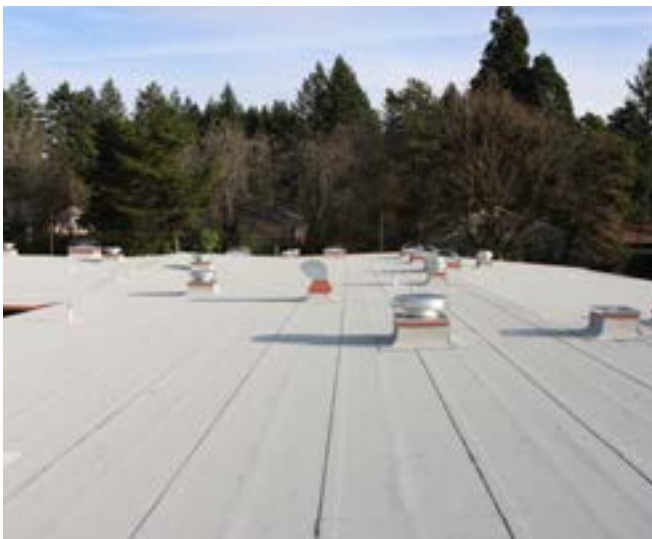
West Sylvan Middle School - New Roof, December 18, 2023
