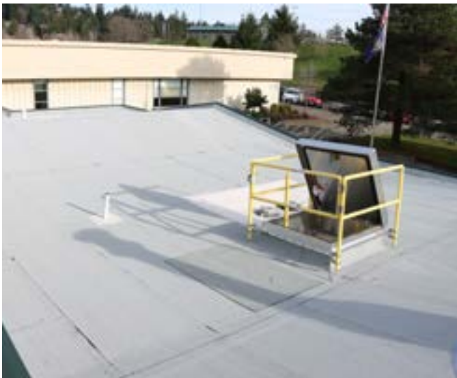
Rieki Elementary School - New Roof, December 18, 2023
