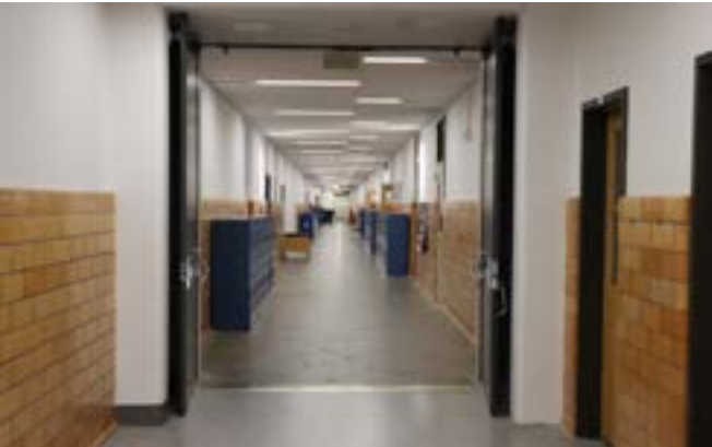
Harrison Park Middle School - Conversion Hallway, March 4, 2024
