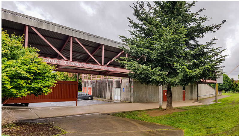
Harriet Tubman Middle School exterior.
