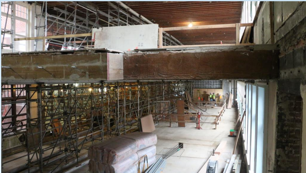
Temp Supports Coming Down
