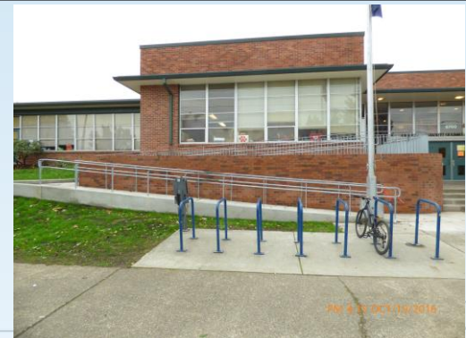
New ADA Ramp at Scott
