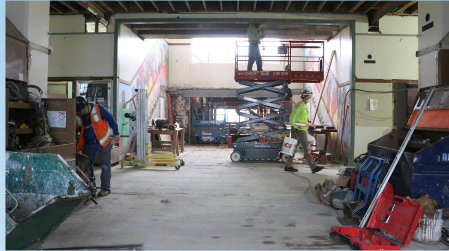
Main Lobby Modernization
