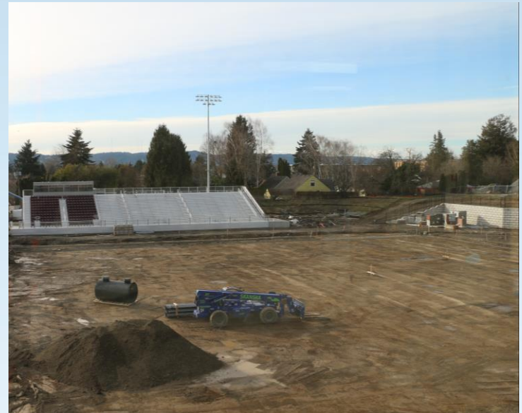
Football Field and Track Under Construction
