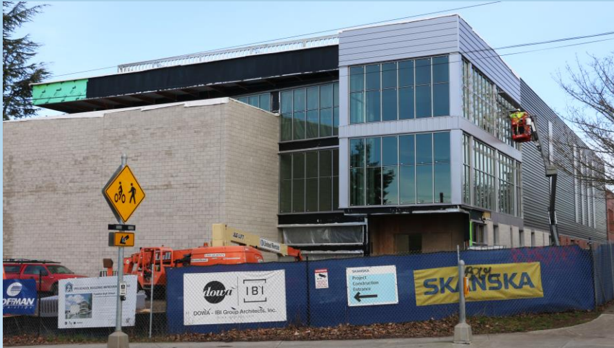
Performing Arts Wing at Corner of 52 nd and Woodward
