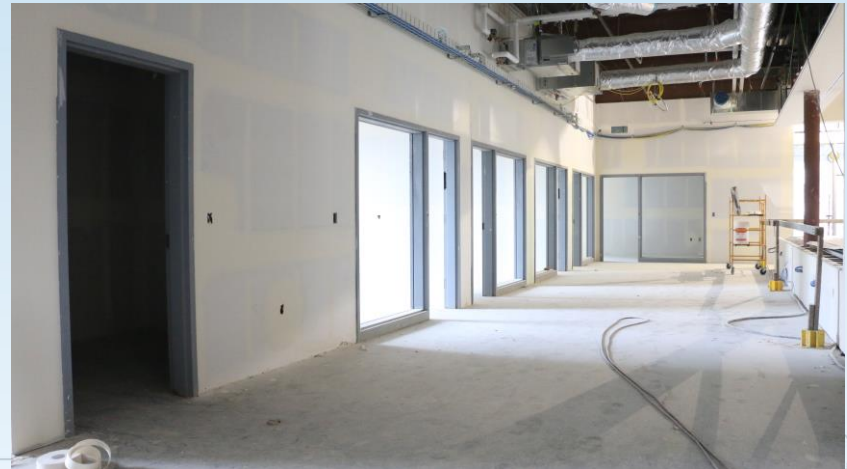
Prep for Paint – South Wing
