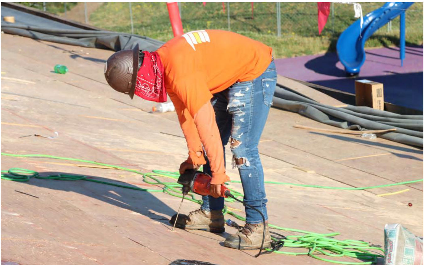
Reike Elementary Roof Project, July 26, 2022
