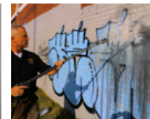
Rinsing larger graffiti after applying BBSM
